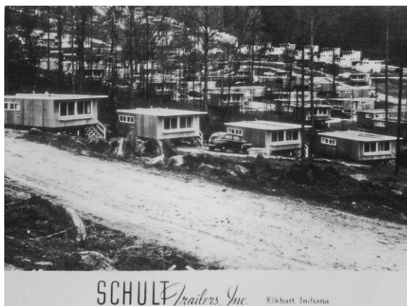
Always an innovator, Schult introduced steel frames, forced air heating, complete interior plumbing and built-in appliances. That was by the forties. During the war, they built 2,000 twin section homes for the Tennessee Valley Authority. A cluster of them adorns the Tennessee hillside above. Bob Richardson helped hammer some of these together for the war effort. Courtesy RV/MH Museum
