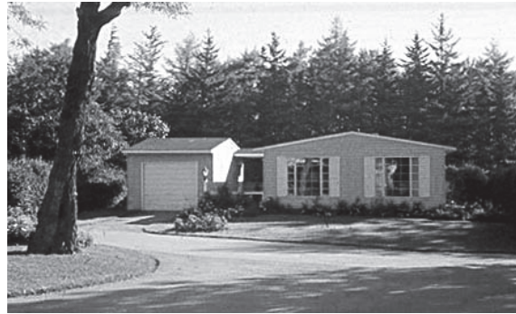
Here's one installed on site.
