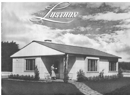
The whole house was delivered on a single semi-trailer and was to be erected on site in jig time.
