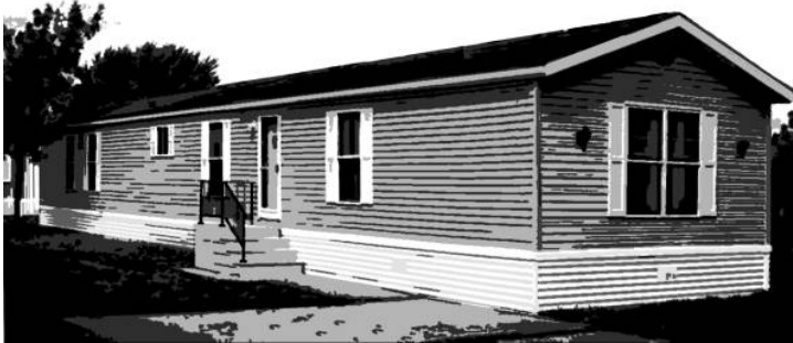
The 16 x 80 MH at left is typical of today's singles. All residential materials—no shiny tin—so why does the market still perceive it to be a homely house? Think about it. No stick builder creates homes of this shape, and such "odd" proportions can't be hidden behind shutters and shingles.
